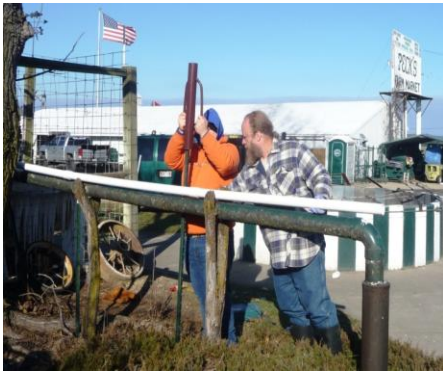
Replacement of an ascending water pipe (green) to a decending water pipe (white) after it was determinend that years of sludge build up supported negative associated organisms in the water.
